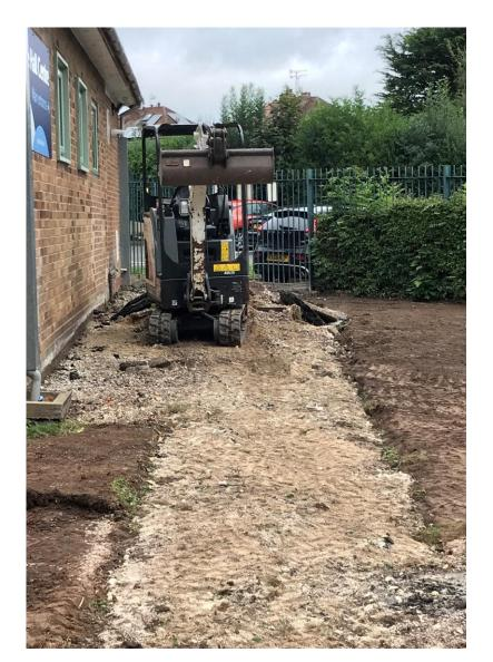
Site levelled with 50 tonne of sub-base to provide a base for fully accessible pathways, planters and ploytunnel.
